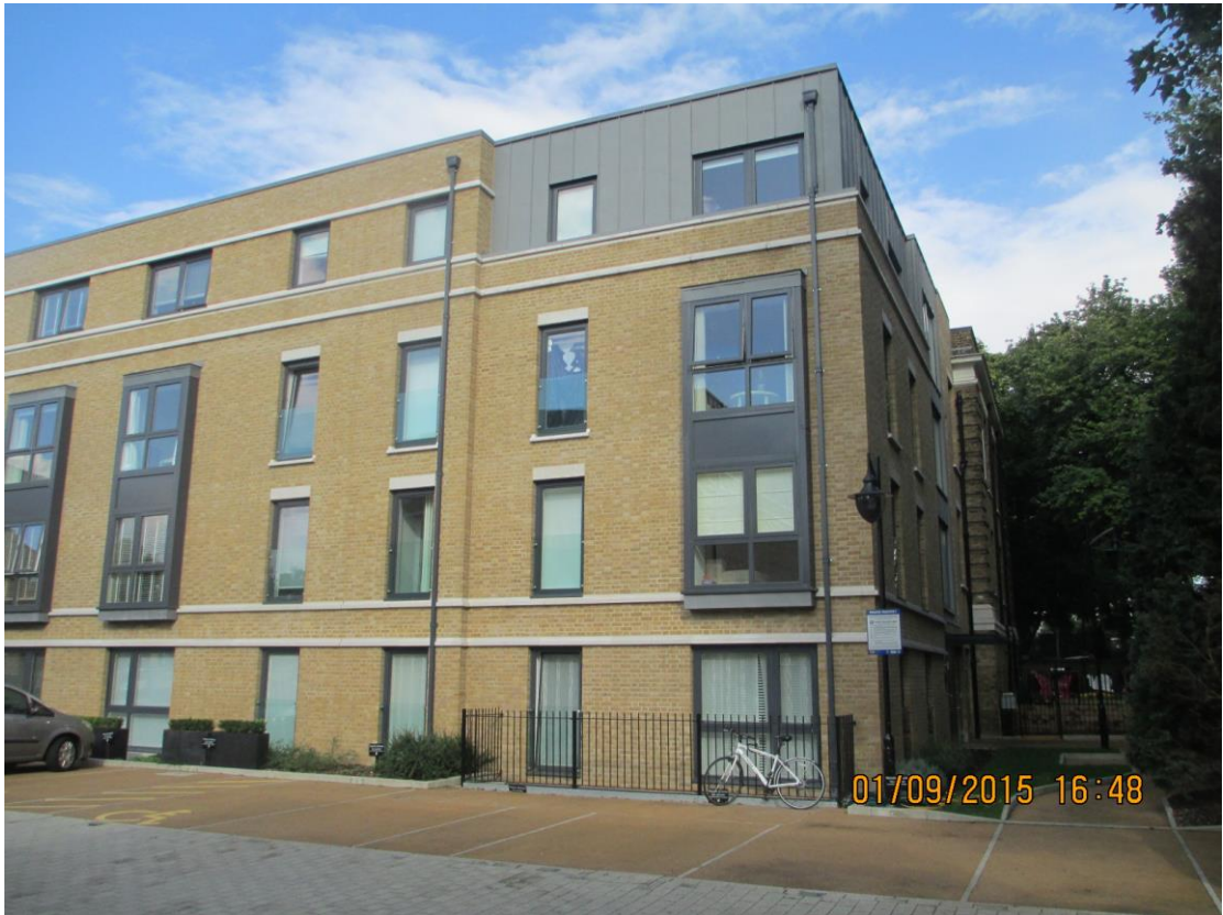
Image 3 – Lightwell in context with existing building.
