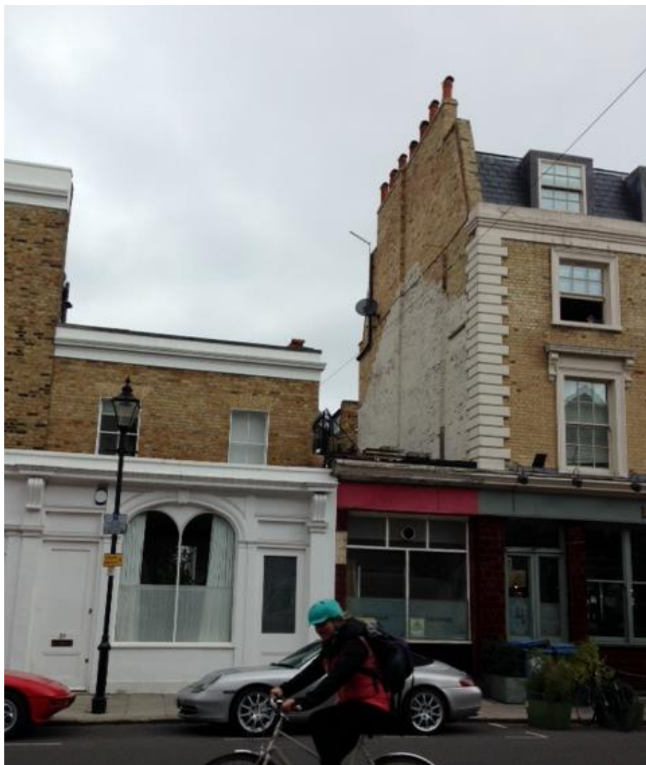
Image 3: view looking at the front façade of 25 Danbury Street
